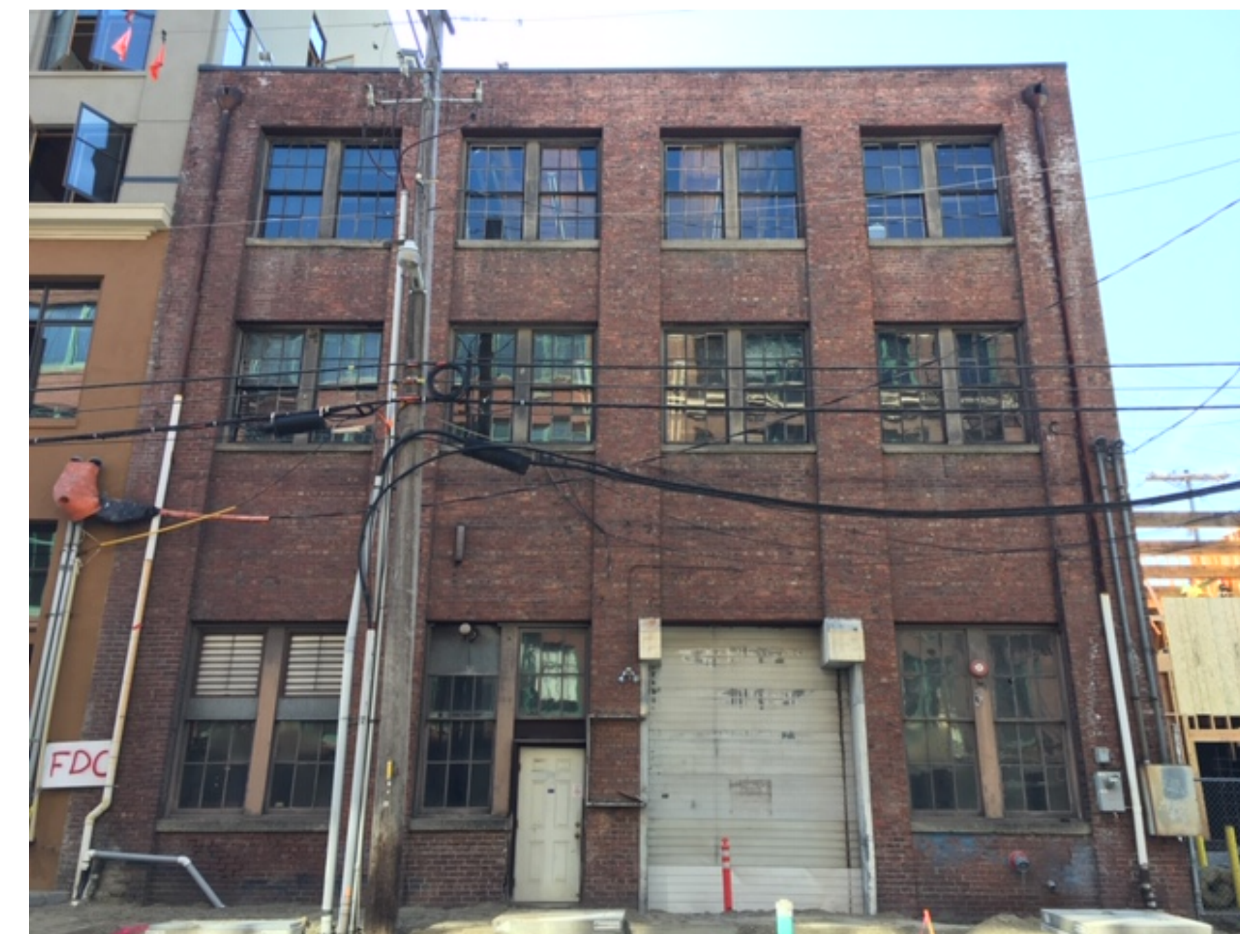
EXISTING COMMERCE STREET FACADE (EAST ELEVATION)
