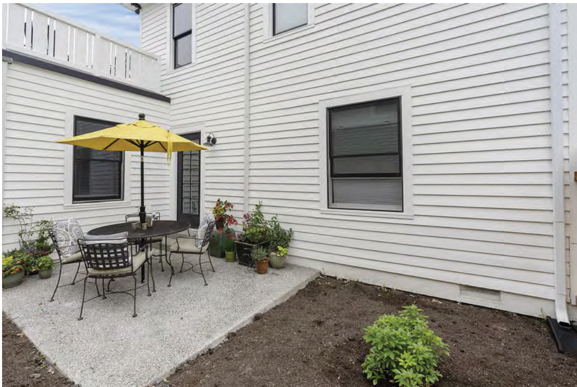
Figure 10. South elevation, looking northwest, 2020.
