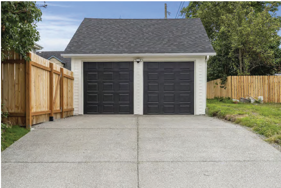
Figure 8. Garage, looking south, 2020.
