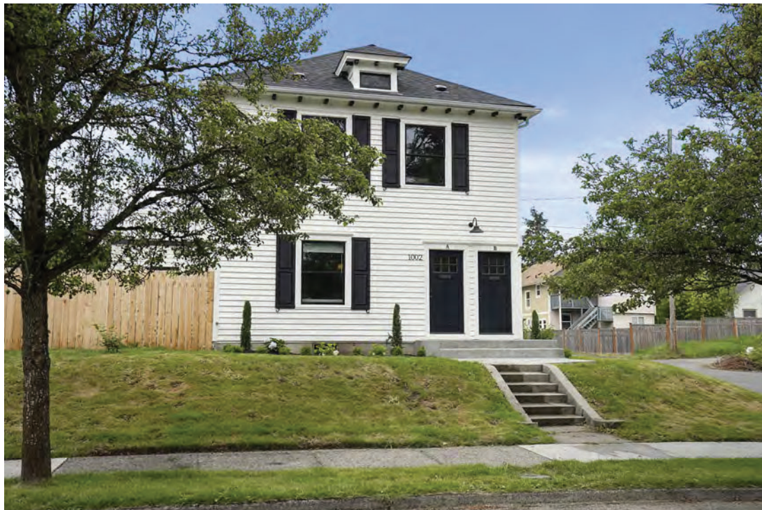
Figure 6. East (main) elevation, 2020.
