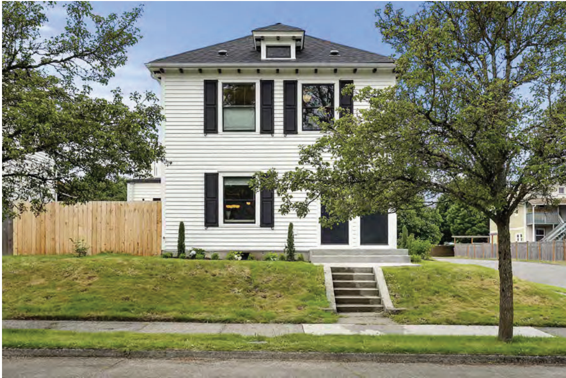
Figure 5. East (main) elevation, 2020.
