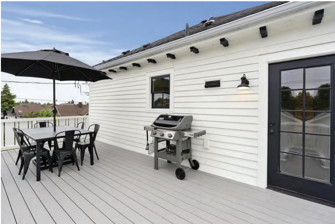
Figure 13. West elevation and 2nd floor deck, 2020.
