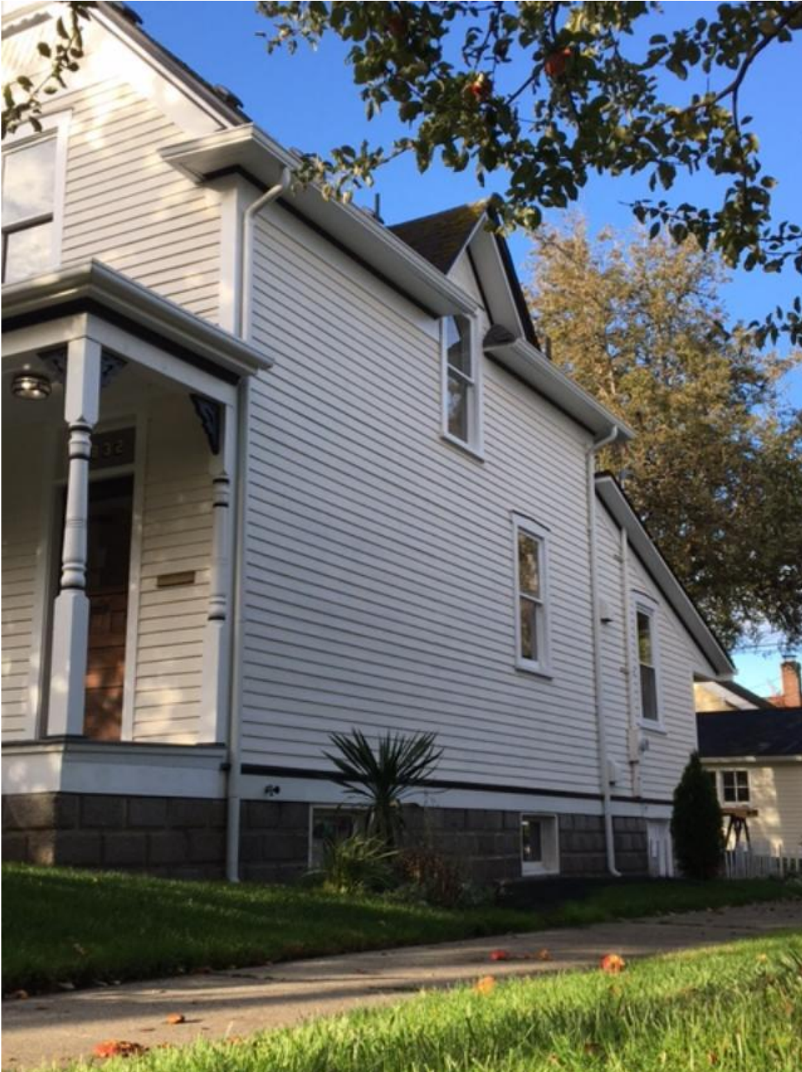
Figure 15. North Façade, 2021 (Collection of Scott Armstrong)
