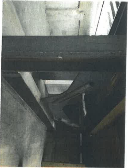
Before – Mezzanine cross-bracing
