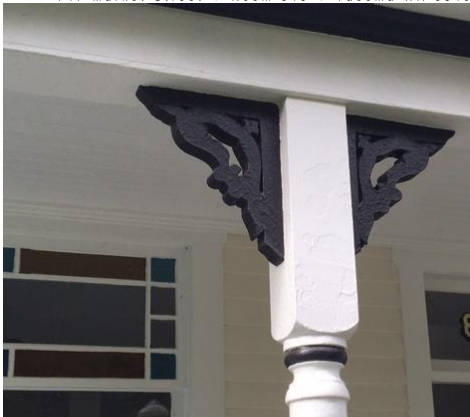
Figure 12. Spindle work brackets, front porch (Collection of Scott Armstrong)
