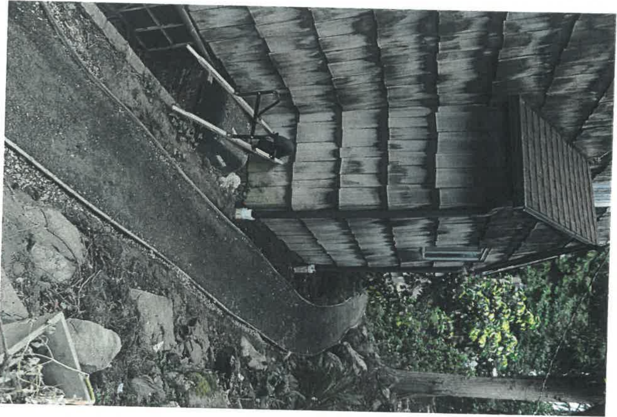
Before Remodel - Siding and Roof
