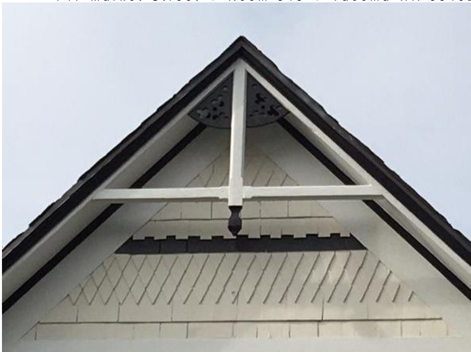
Figure 10. Main, front gable decorative “collar tie with drip” truss in the pitch and dormer gable clad in alternating sections of staggered-butt and saw-tooth wood shingles. (Collection of Scott Armstrong)
