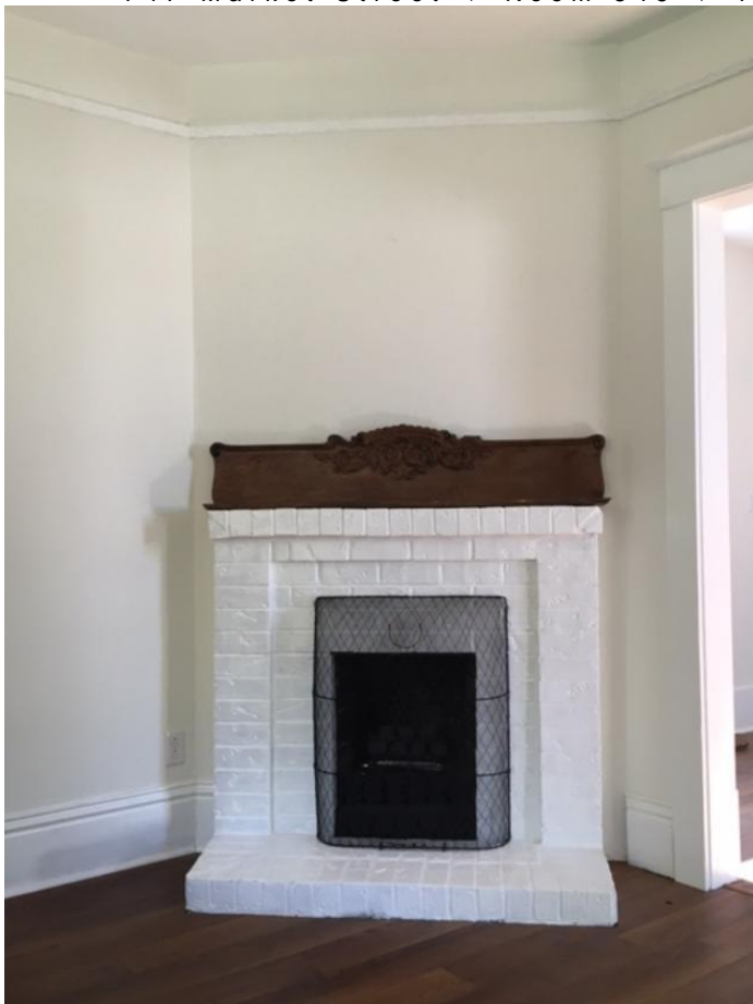
Figure 19. Front parlor; coal-burning fireplace with original cast iron coal basket, grate, and screen (Collection of Scott Armstrong)
