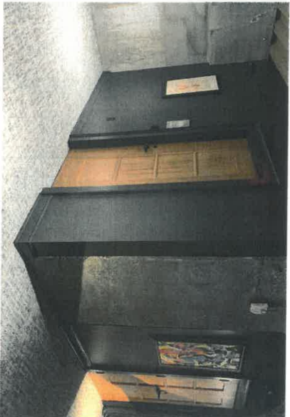
After – Mezzanine, looking toward restroom
