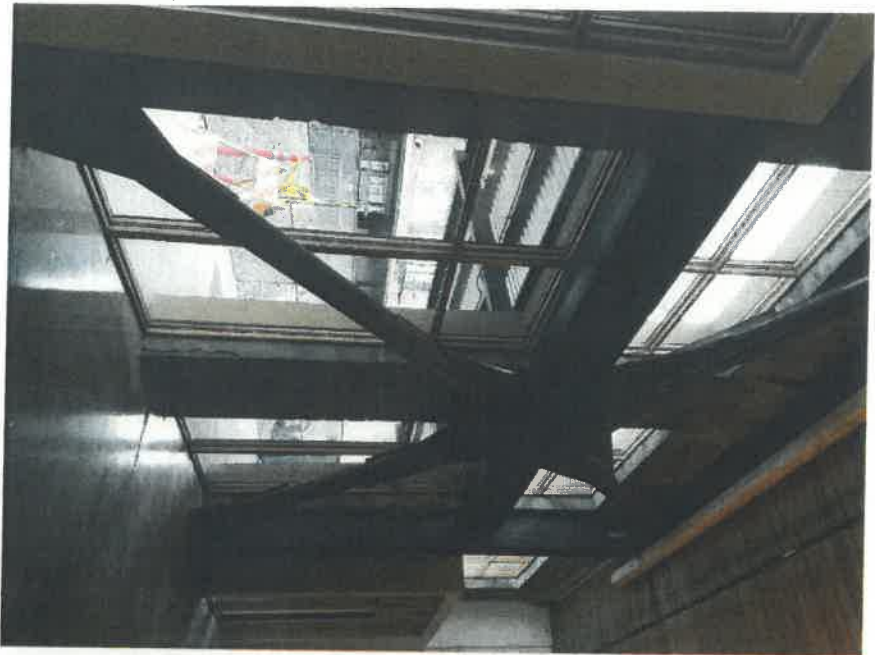
Before – Cross-bracing at exterior wall
