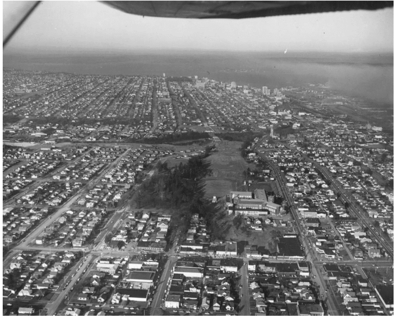
1961 aerial view of Lincoln neighborhood, looking north. Source: Tacoma Public Library, image Richards Studio D129752-1.
