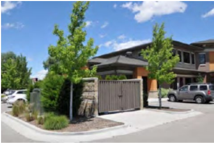
Well-designed service enclosure example.
