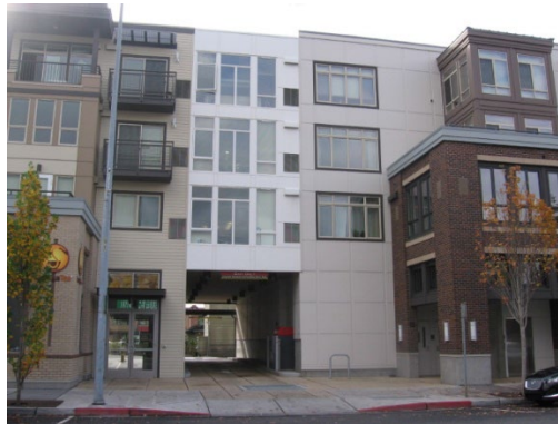
Example of a drive-through within a structure
