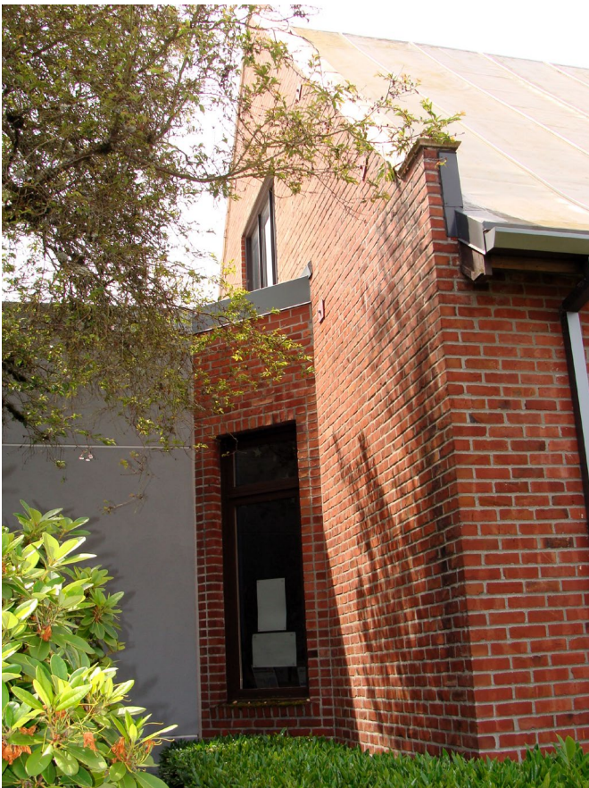
Figure 20. Anna E. McCormick building, east façade, 2024. Note that the 1927 bay remains intact while the 1959 addition is now clad in gray stucco as the connection with the new Wheelock building.
