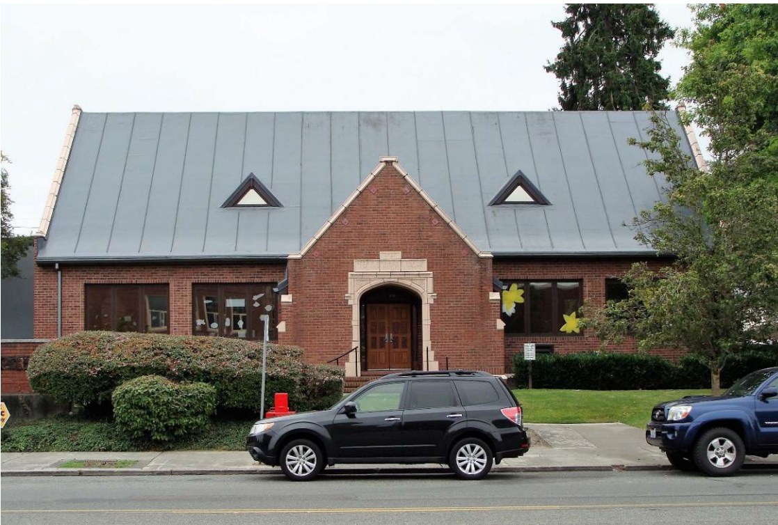
Figure 18. Anna E. McCormick building, front (north) façade, 2019
