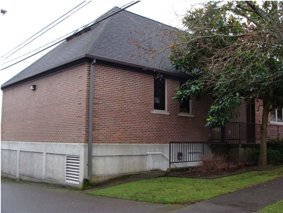
Figure 17. Northeast (front) corner of the north wing of the Mottet Library (McClintock, 2021)
