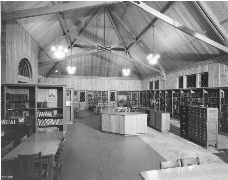
Figure 7. Original interior of Mottet Library showing the western hemlock interior. (Tacoma Public Library, BU-10242)
