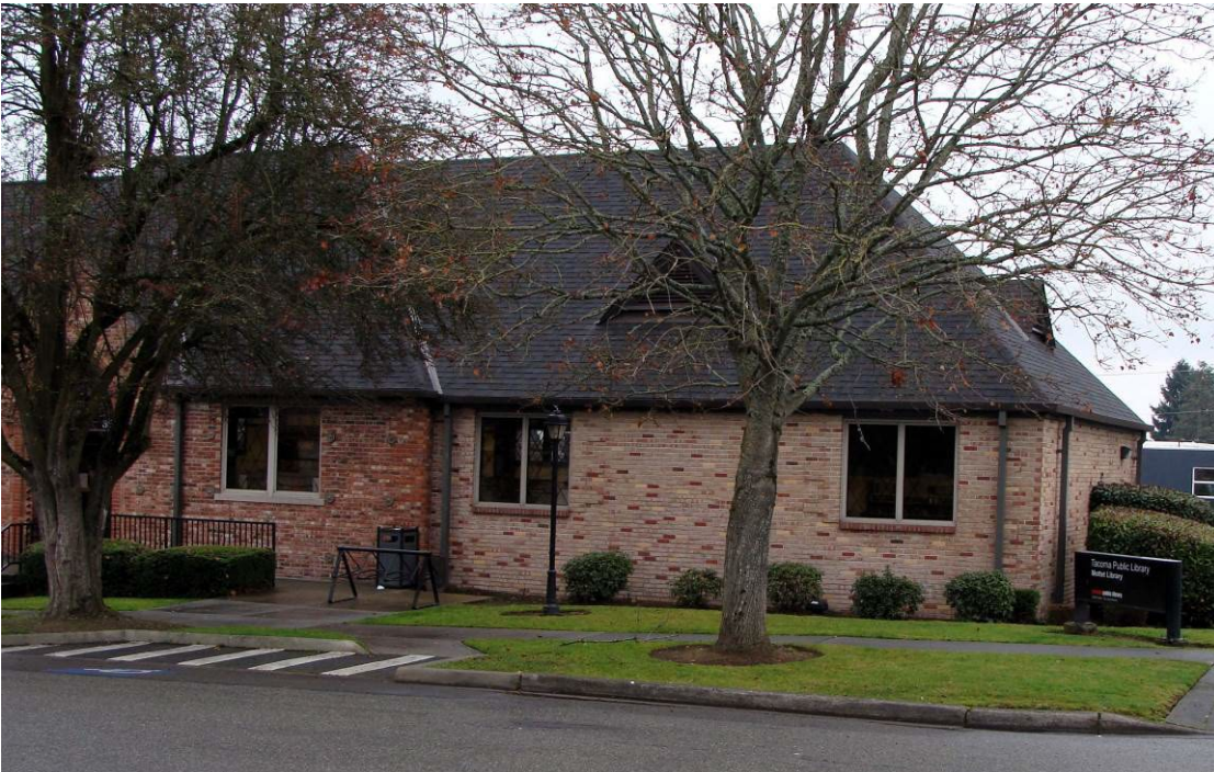
Figure 14. Front façade of the south wing of the Mottet library. (McClintock, 2021)
