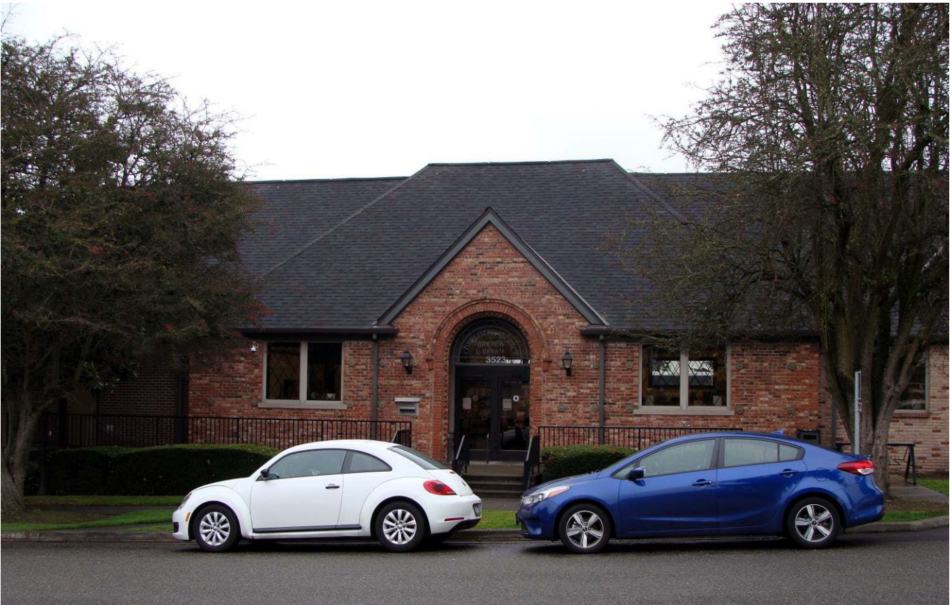
Figure 12. The central section and main entrance of Mottet Library. (McClintock, 2021)
