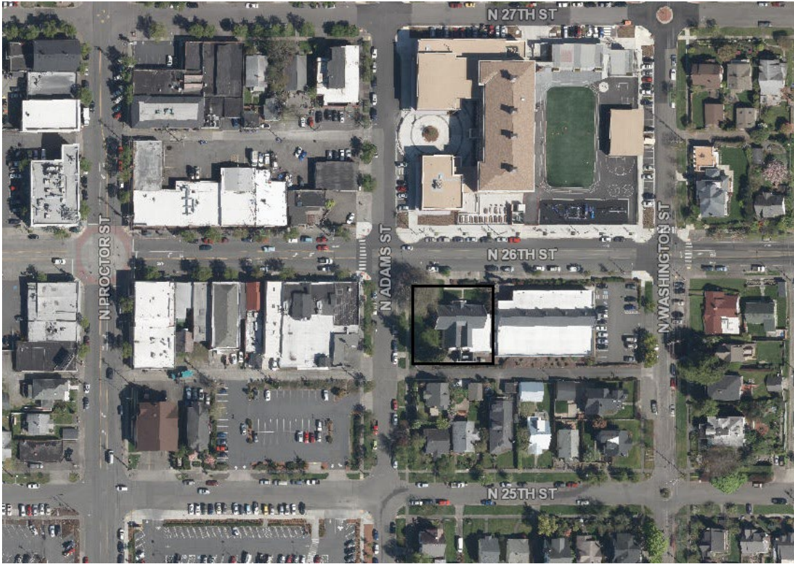
Figure 1. Aerial neighborhood view. Nominated property outlined in black.
