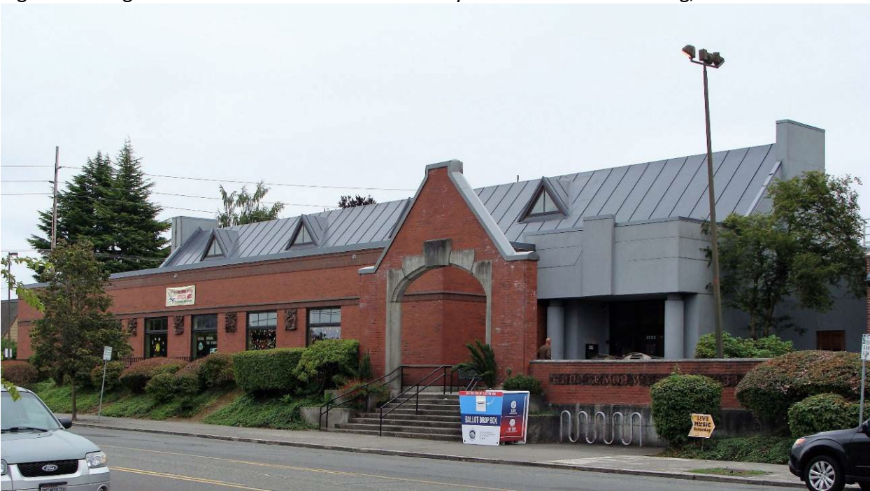
Figure 23. Virginia Lemon Wheellock Branch Library, the 1988 addition, 2019
