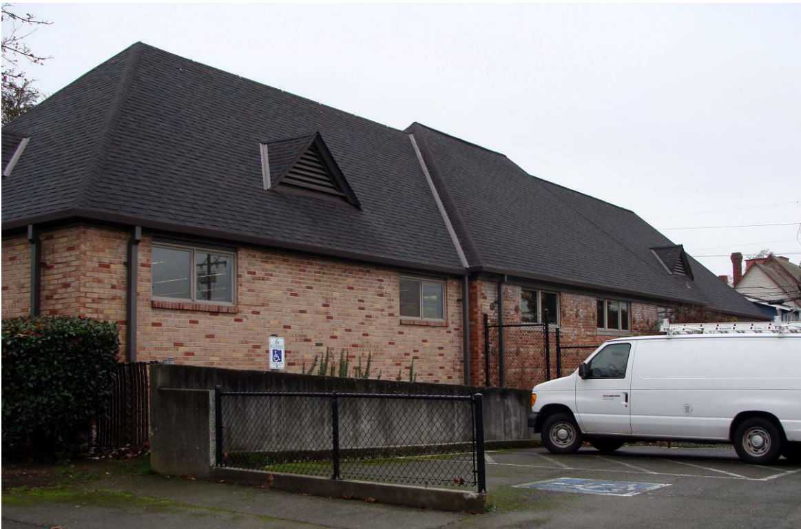
Figure 16. West (rear) façade of the Mottet Library (McClintock, 2021)
