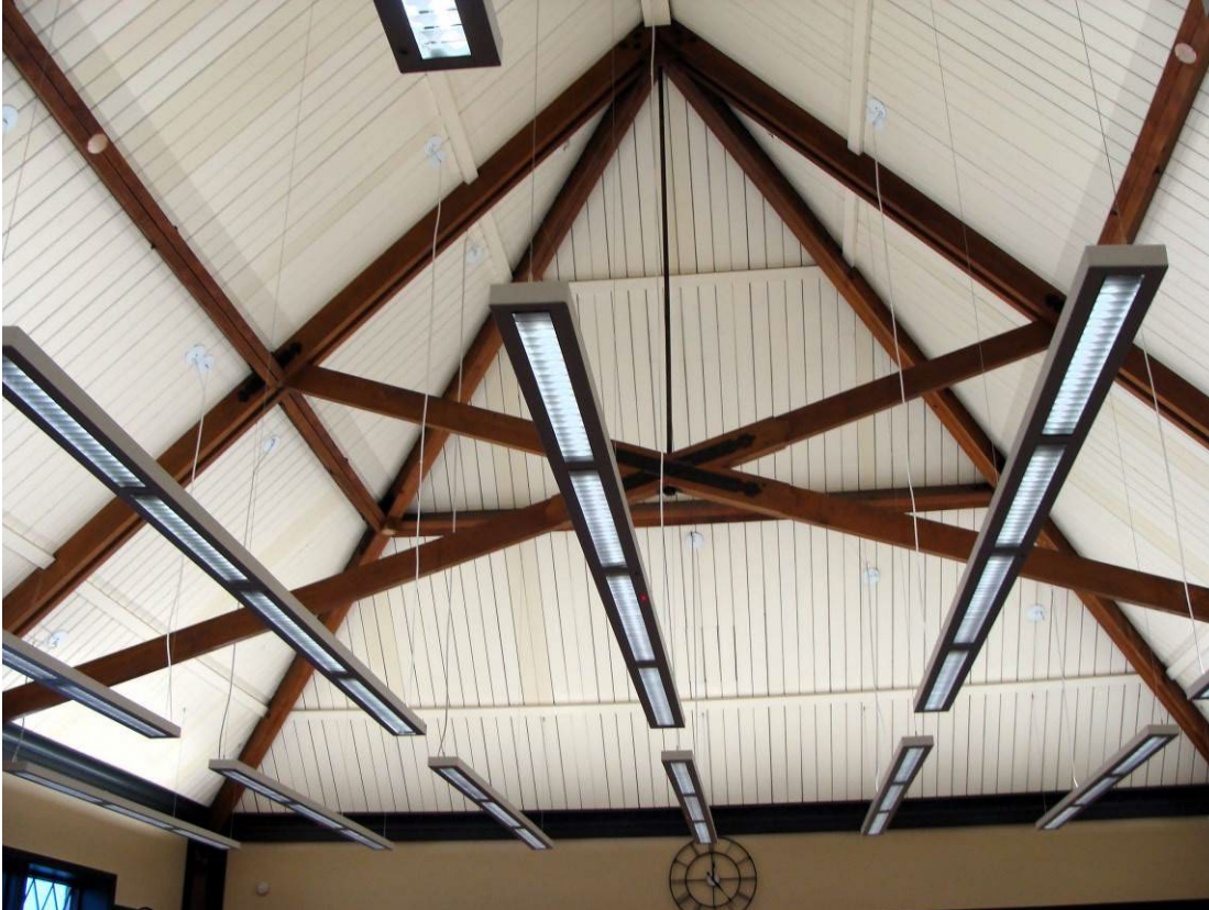
Figure 19. Interior of the Mottet Library showing the vaulted ceiling and trusses. (McClintock, 2021)
