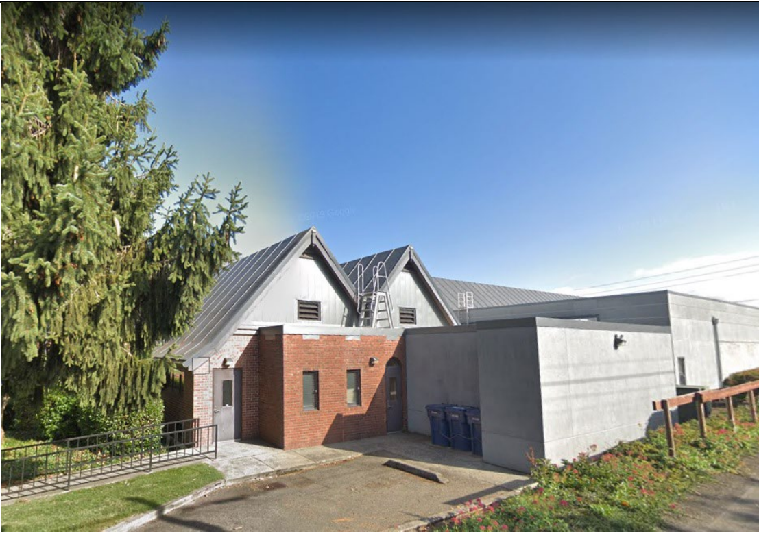
Figure 20. Anna E. McCormick building, southwest rear façade. Brick section is the 1959 addition. 2019
