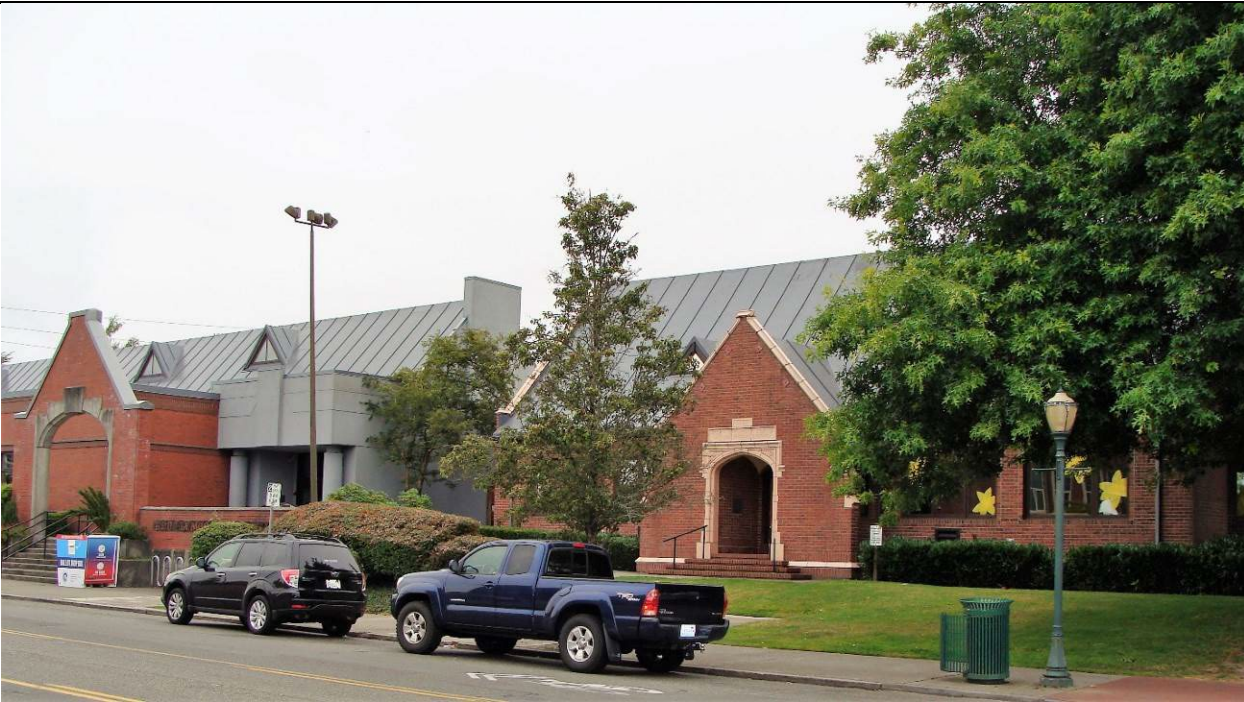
Figure 22. Virginia Lemon Wheellock Branch Library and McCormick building, 2019
