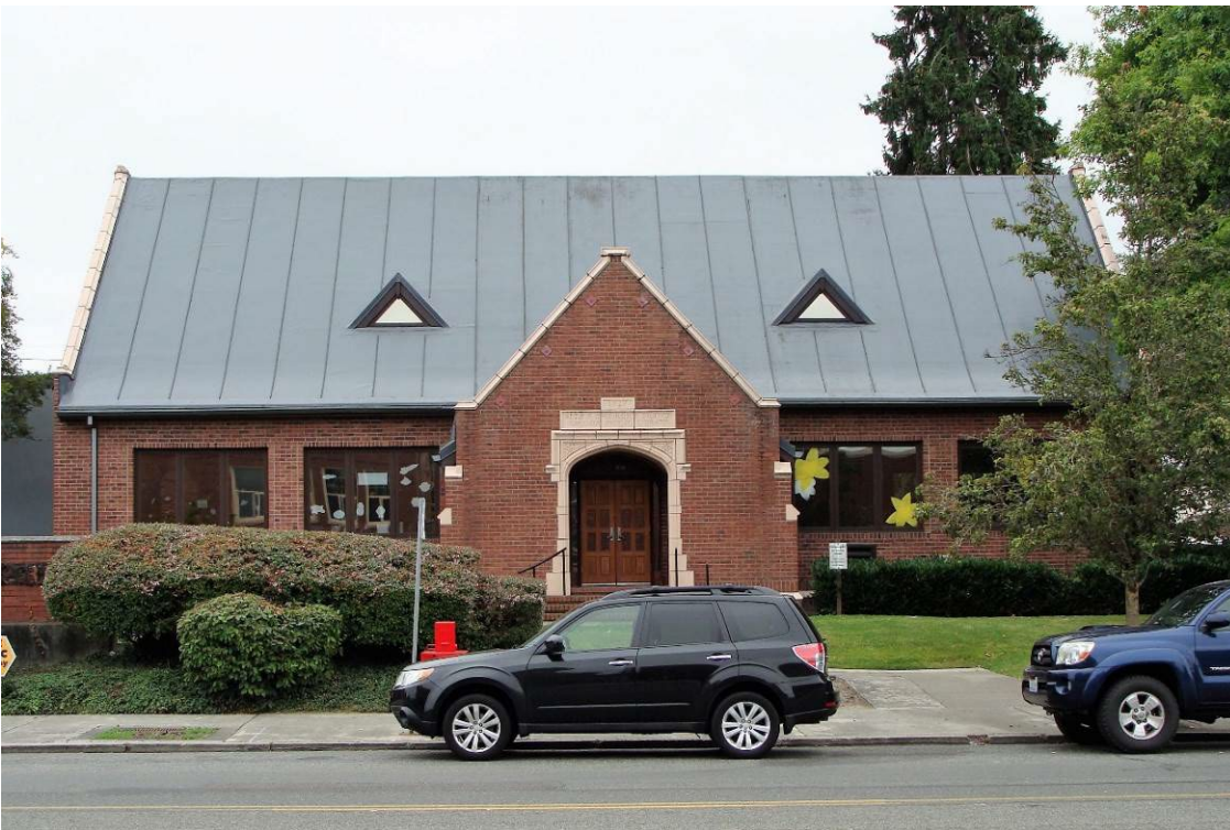
Figure 18. Anna E. McCormick building, front (north) façade, 2019
