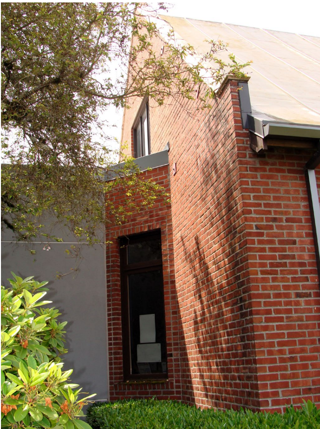
Figure 20. Anna E. McCormick building, east façade, 2024. Note that the 1927 bay remains intact while the 1959 addition is now clad in gray stucco as the connection with the new Wheelock building.
