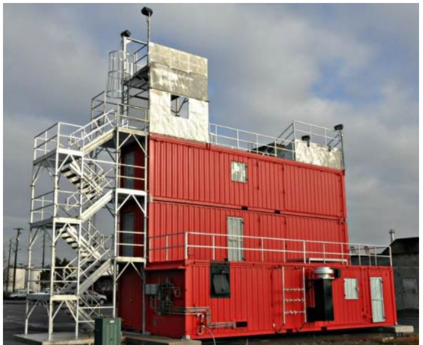
Live-Fire Training Prop – Training Center
