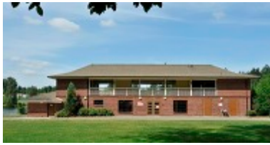
Wapato Park bathhouse, 2024
