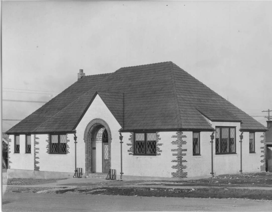
Figure 5. Mottet Library shortly after construction. 1930. Note the whitewashed brick. (Tacoma Public Library, BU-10241)
