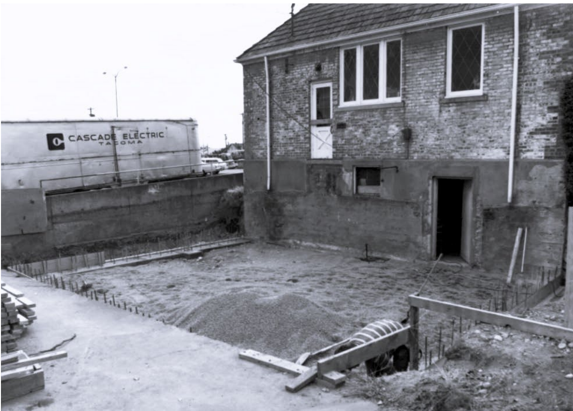
Figure 10. Excavation for expanded north wing, 1977 (Tacoma Public Library, BU-14228)
