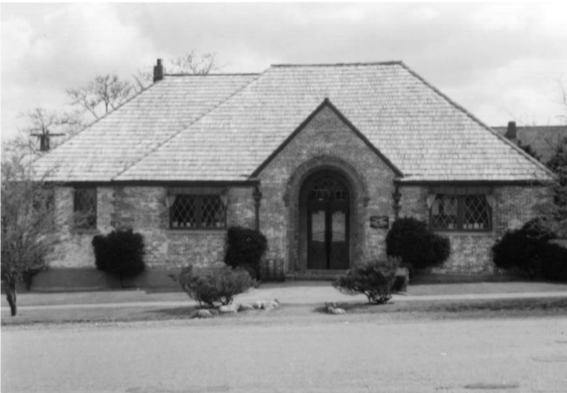
Figure 6. Mottet Library about 1960 showing original north wing and whitewash removed (Tacoma Public Library, BU-11855)
