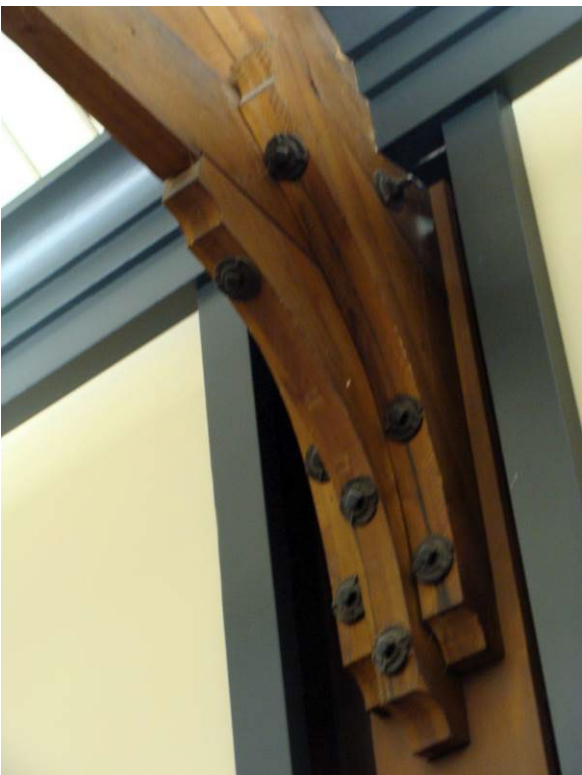
Figure 20. Detail of original truss connection, Mottet Library, (McClintock, 2021)
