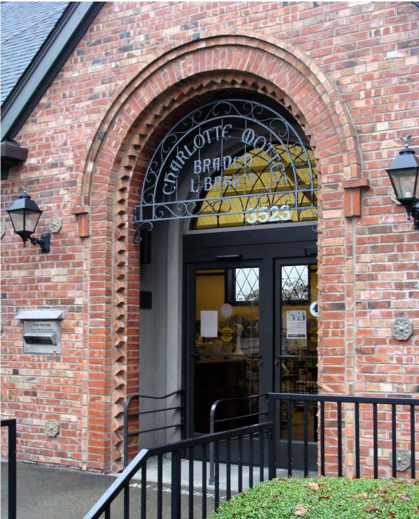
Figure 13. Detail showing the elaborate brickwork of the entry, Note the round earthquake bolts. (McClintock, 2021)
