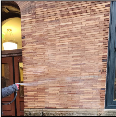
8:15 AM Low-pressure, water rinse using spray nozzle.
