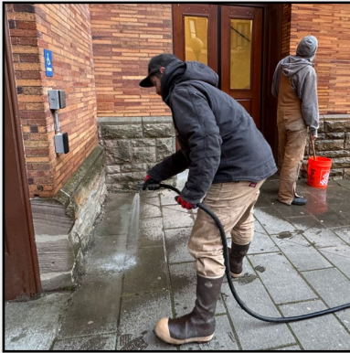
8:15 AM Low-pressure, water rinse using spray nozzle.
