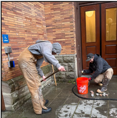
8:25 AM Vana Trol application using natural bristle brush. Approximately 22 minute dwell time.
