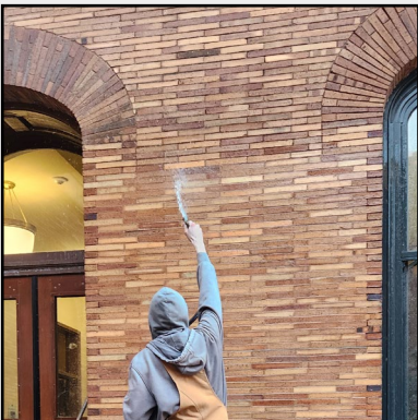
8:40 AM Low-pressure, water rinse using spray nozzle.
