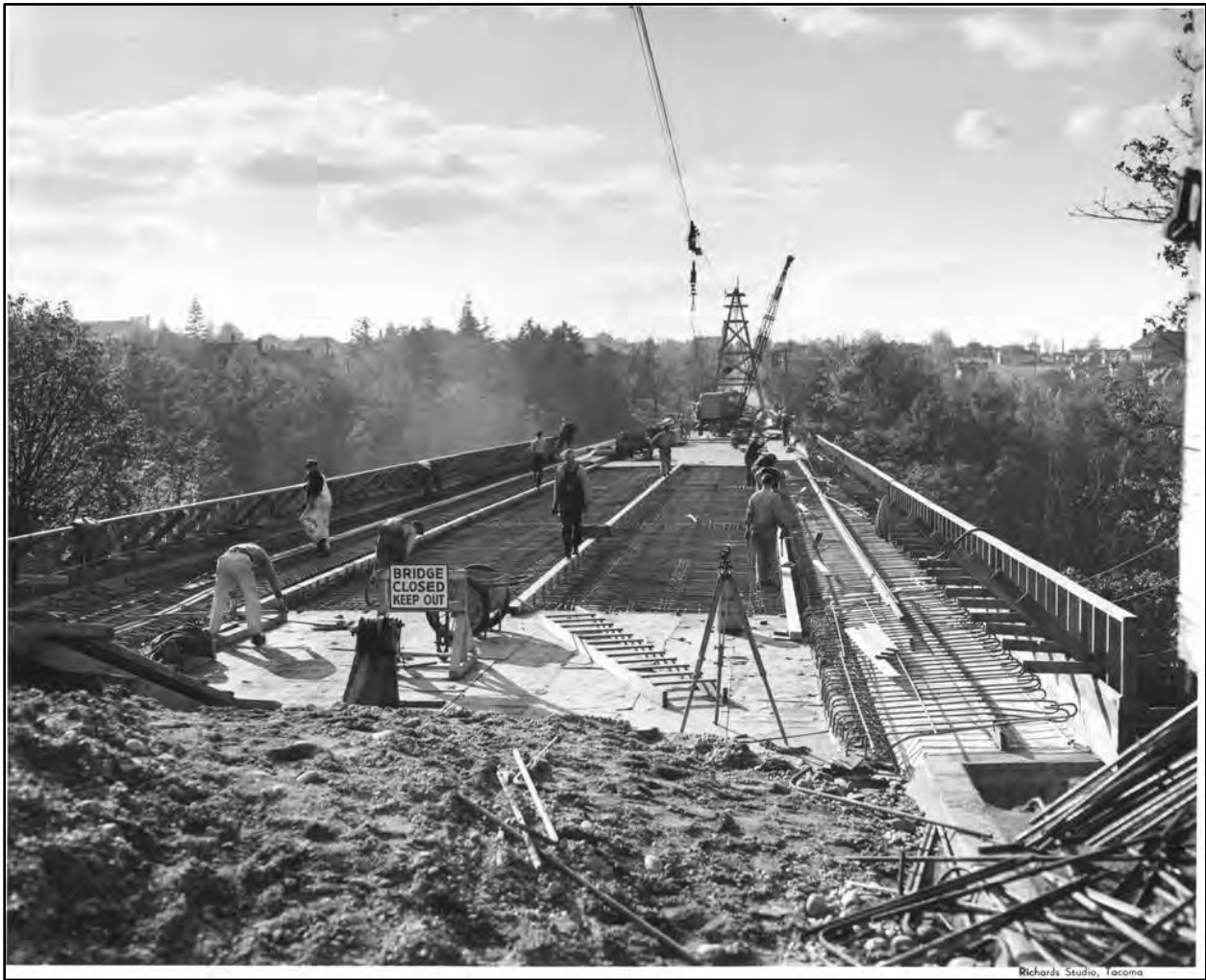
Figure 26. The in-construction phase of East 34th Street Bridge – Pacific to A Street circa 1935 (Tacoma Public Library 2024).
