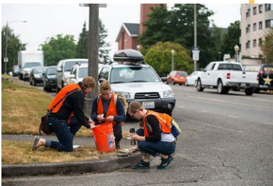
Volunteers attach “No Dumping, Drains to Puget Sound” markers next to storm drains
