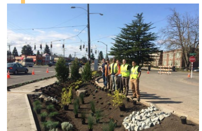
Volunteers replace asphalt with plantings along Division Ave and Sprague Ave to compliment the City's adjacent new rain garden
