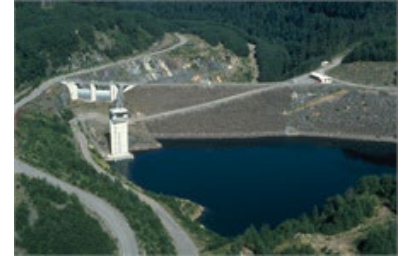
Howard Hanson Dam
