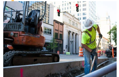
Construction on Pacific Ave
