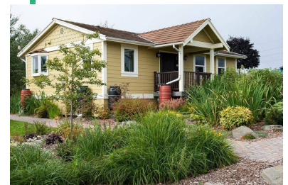
EnviroHouse, a permanent model home showcasing green building and natural landscape ideas, located at the Tacoma Landfill
