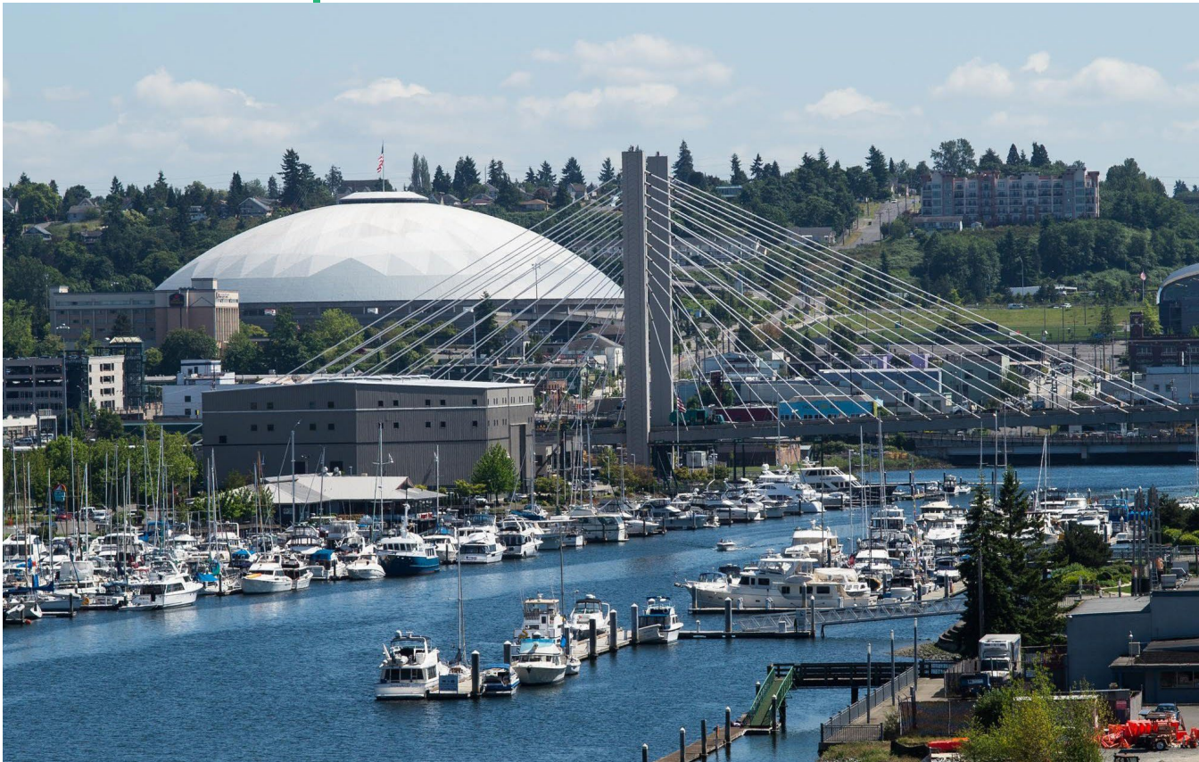
View of the Tacoma Dome and SR 509 cable-stayed bridge crossing the Thea Foss Waterway
