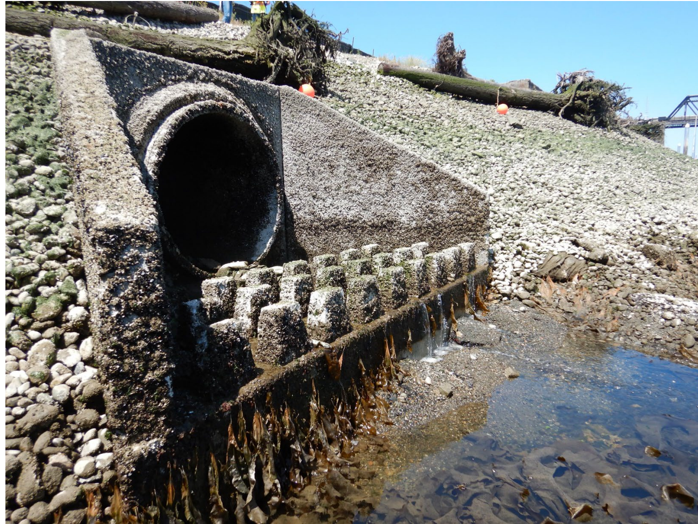
Photograph 1. City Outfall 230A outlet to the Thea Foss and Wheeler-Osgood waterways west bank during the Year 17 low-tide slope cap inspection as part of the Long-Term Monitoring Plan (LTMP) taken at -3.1 feet mean lower low water (MLLW). Loss of slope cap material, round river cobbles, placed off the outfall apron exposing gravel and sand below top ledge of the apron.
