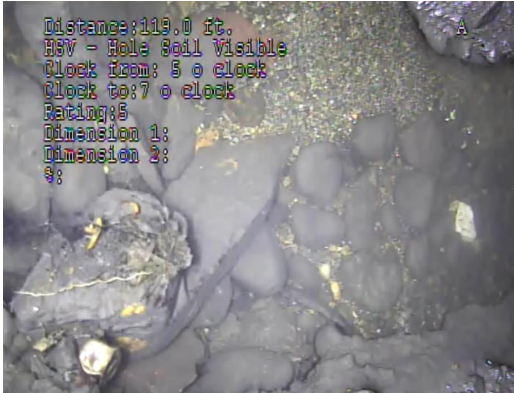
Spot Repair Liner from 119 LF Upstream to 122 LF Upstream
