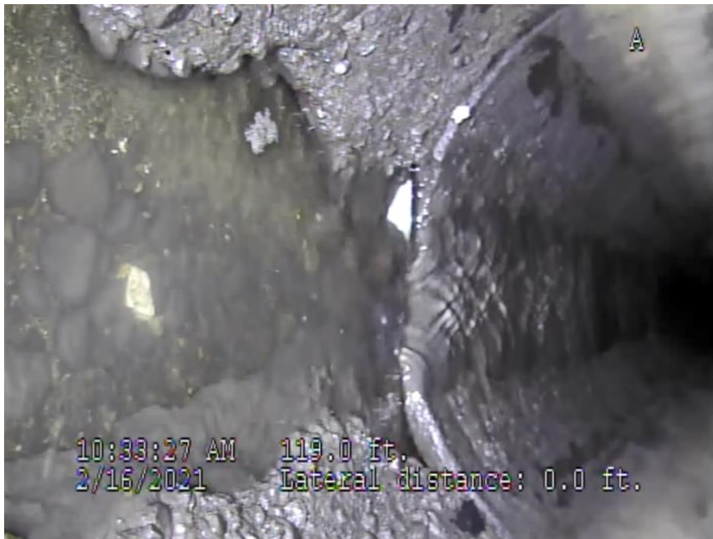
Spot Repair Liner from 119 LF Upstream to 122 LF Upstream
