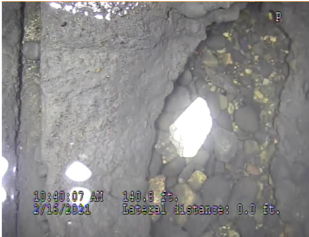
Spot Repair Liner at 140.8 LF Upstream for missing bottom of pipe
