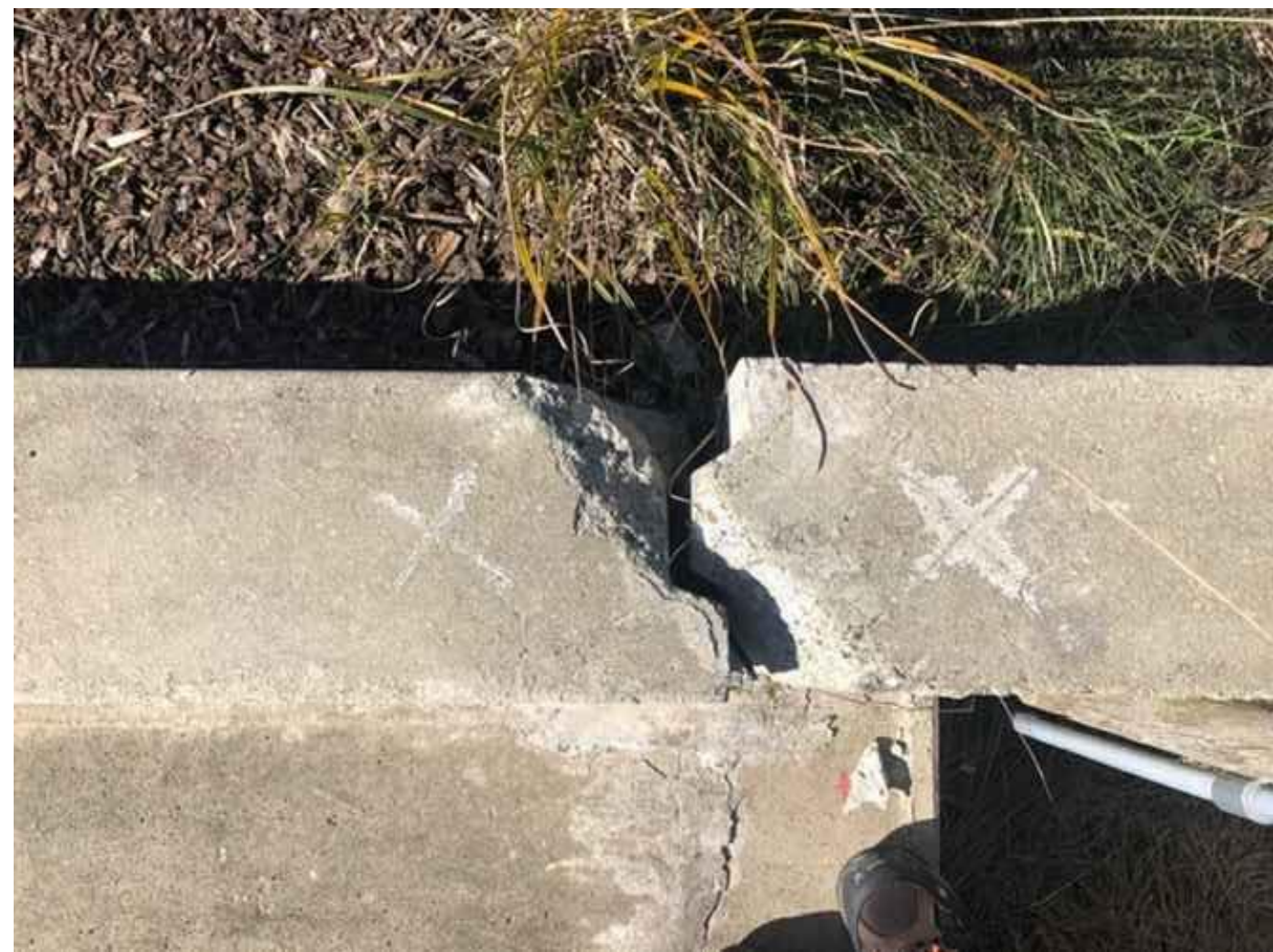
Figure 5: Survey Marks at Joint
