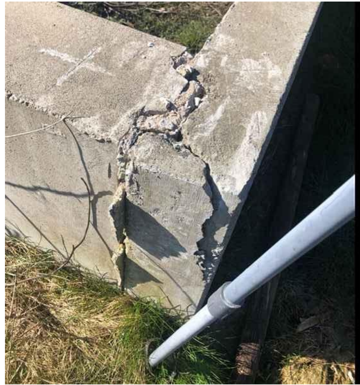
Figure 3: Corner Spall
