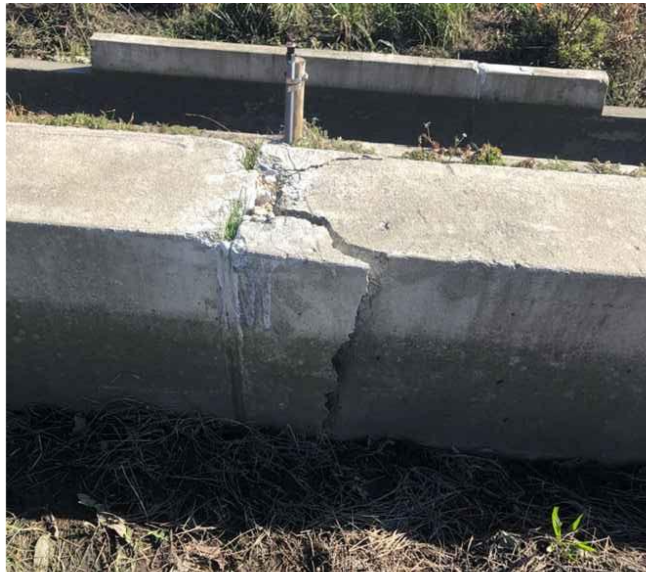
Figure 4: Joint Waterstop
