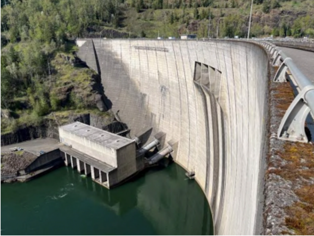
Looking to Right Abutment
