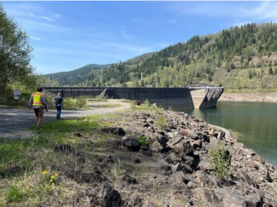
Upstream of Dam looking at Spillway Piers
