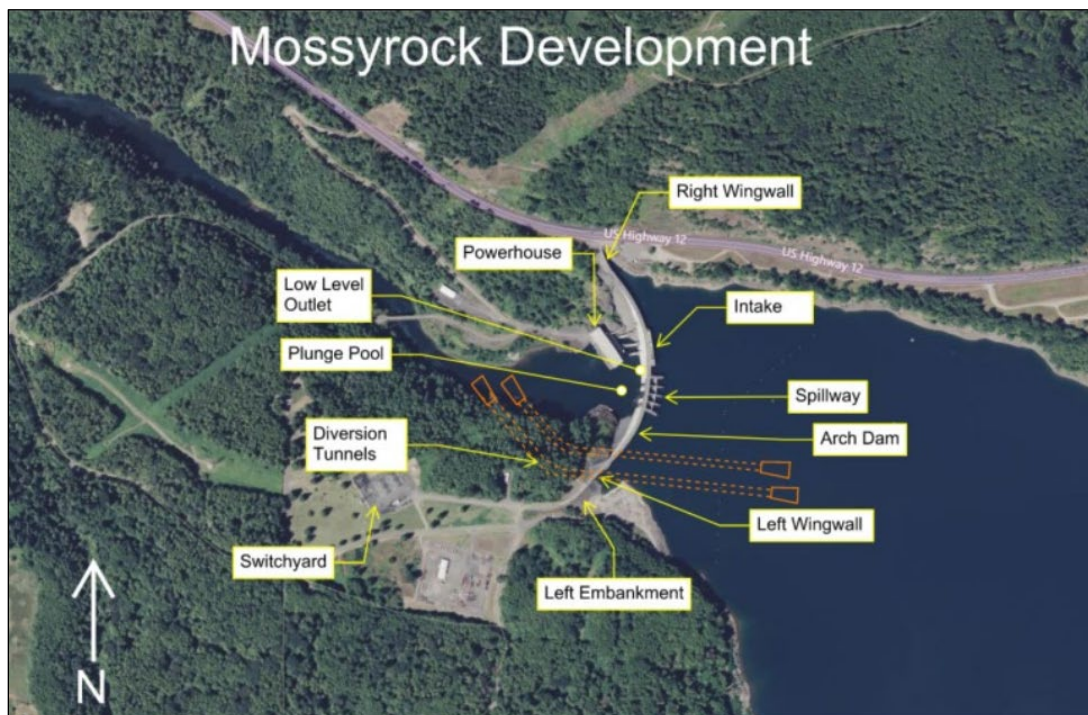
Figure 1 - Overview of Development Structures at Dam Site
