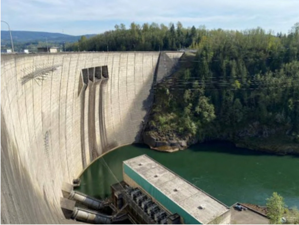
Looking to Left Abutment
