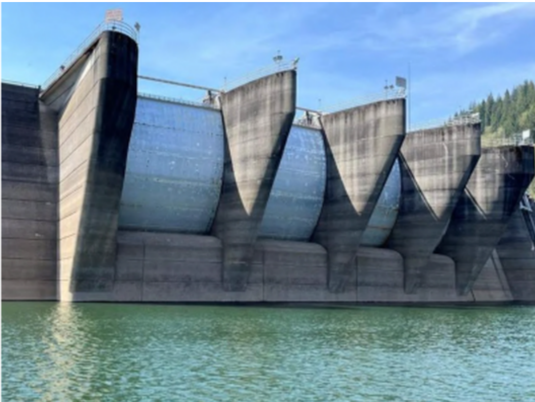
Upstream View of Spillway Piers
