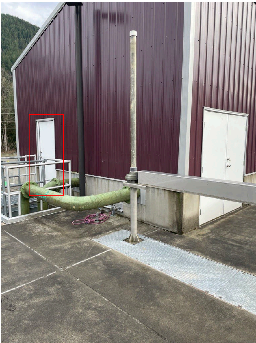
Upper Deck of Flash Mix: Temporary Connection for LA and PACL
