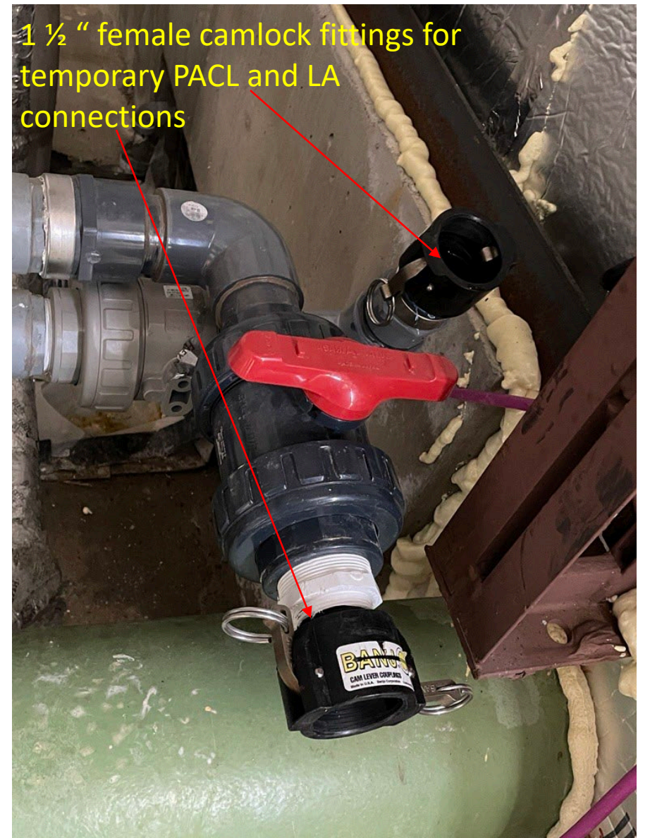
Upper Deck of Flash Mix: Temporary Connection for LA and PACL
