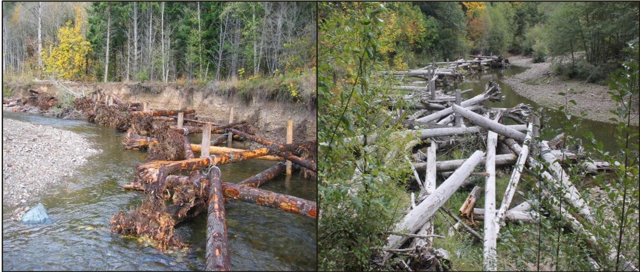
Figure 2. Fish habitat project known as an engineered log jam, located near river mile 85. Left picture taken soon after construction in 2005 (looking downstream), right picture after 10+ years of decay in 2017 (looking upstream).
