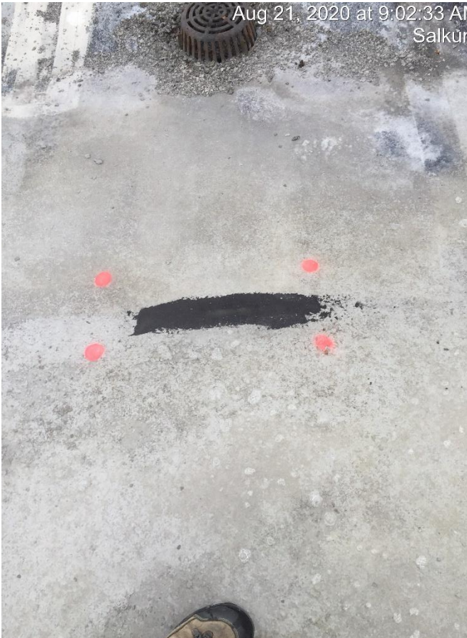
Henry's 208 Wet Patch application
