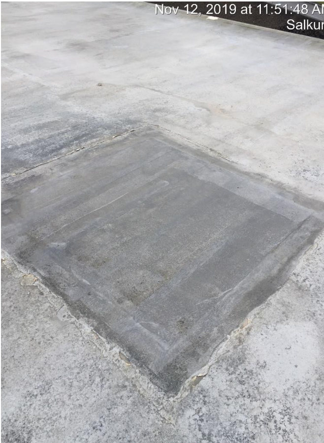
Old equipment repair using Kemper System products
