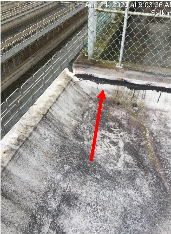
Henry's 208 Wet Patch application
