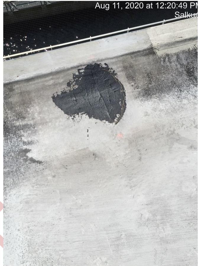
Henry's 208 Wet Patch application
