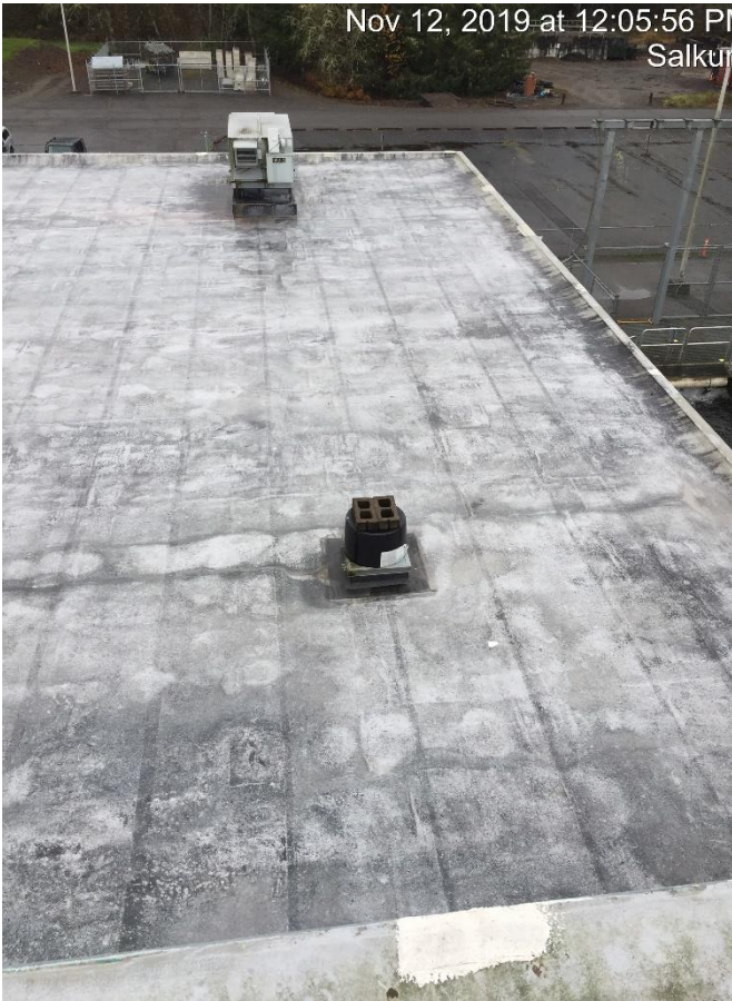
Kemper System-1 piece membrane roof over-coat system (westerly roof)
