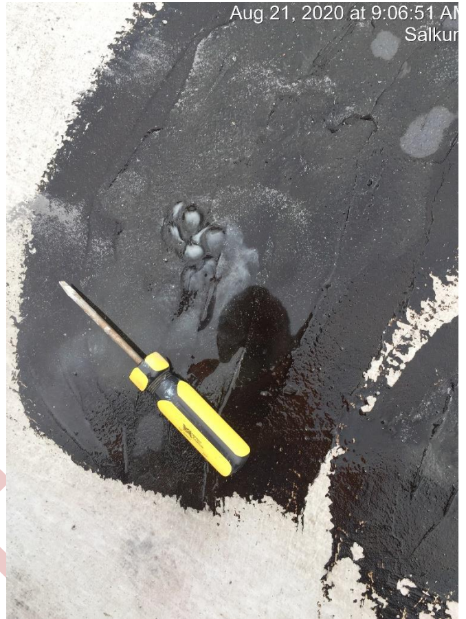
Henry's 208 Wet Patch application
