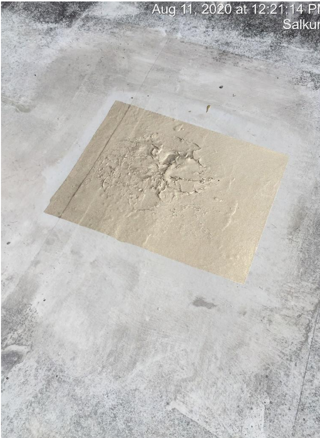
Henry's 555 Fibered Aluminum Coating applied directly over the existing silicone maintenance coating
