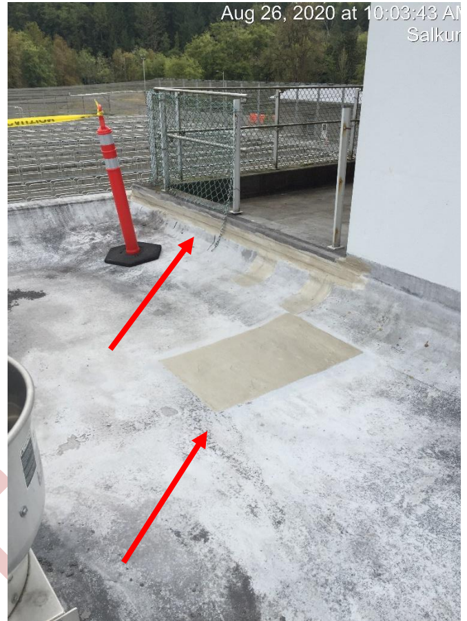
Henry's 555 Fibred Aluminum Coating applied over the Henry's 208 Wet Patch Repair
