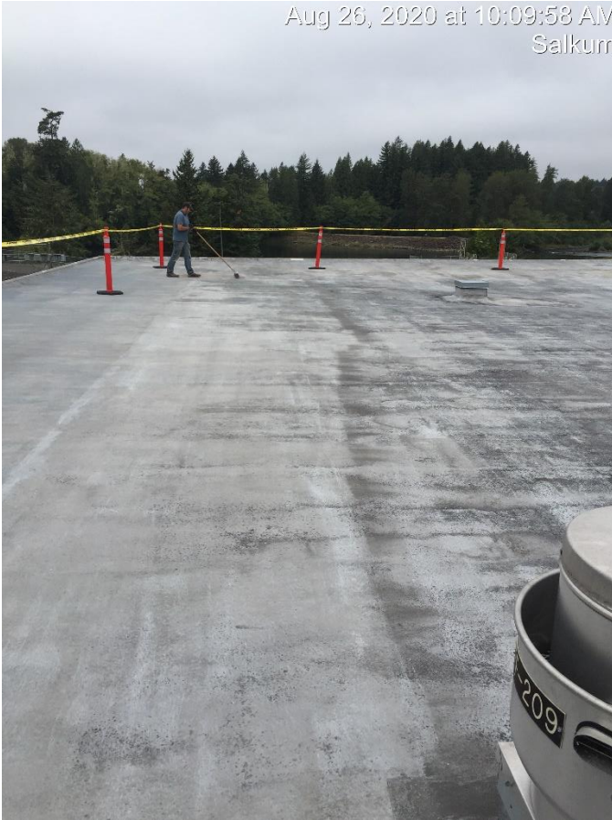
Cowlitz Project Staff cleaning roof sections
