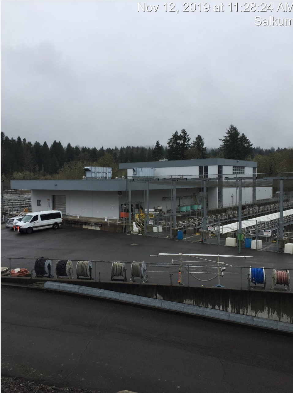
The Cowlitz Salmon Hatchery Early Rearing Building (SH-1)
