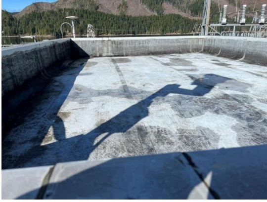
View of Tram House Roof
