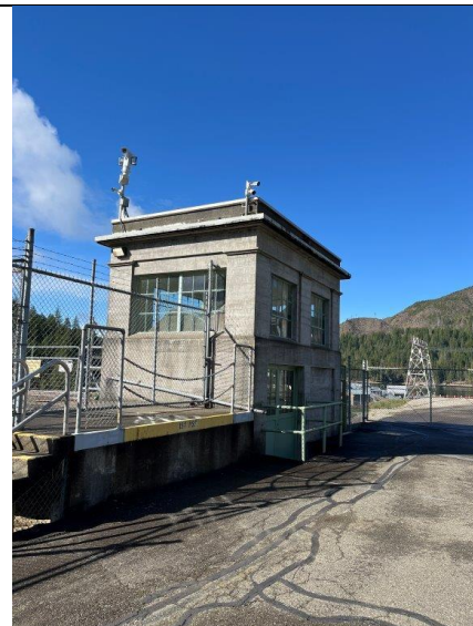
Second View of Cushman 1 Tram House
