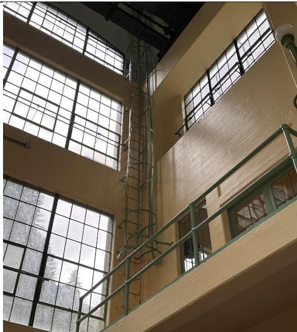
View of Cushman 1 roof access.
