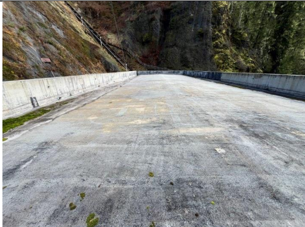
Cushman 1 Main Roof
