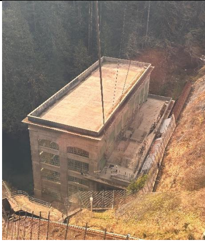
Cushman 1 roof (main roof and annex roof)
