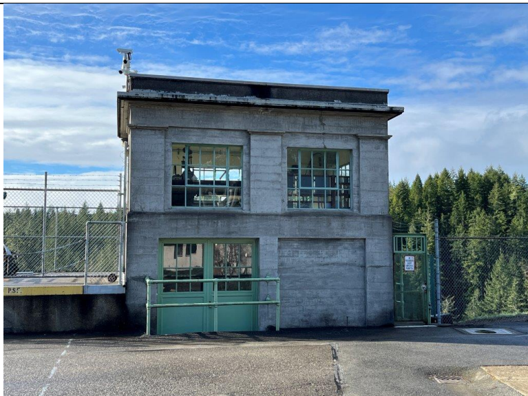
View of Cushman 1 Tram House
