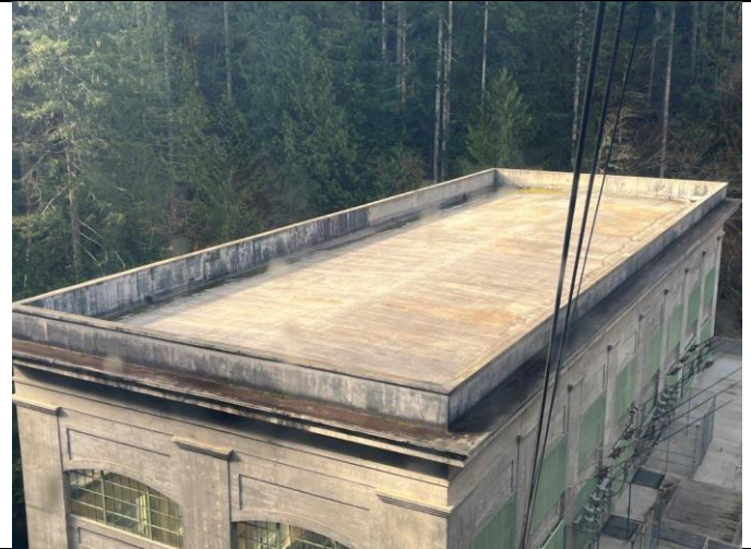
Closer view of Cushman 1 roof
