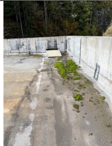
Cushman 1 Main Roof looking at roof access hatch.
