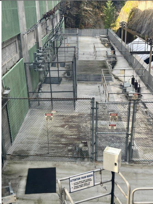
Cushman 1 Annex Roof (note: high voltage along left wall)
