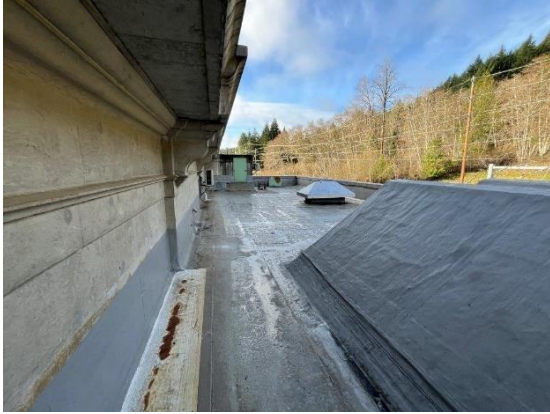
Annex roof looking south
