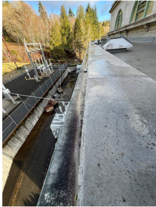
Annex roof overhang and roof vent
