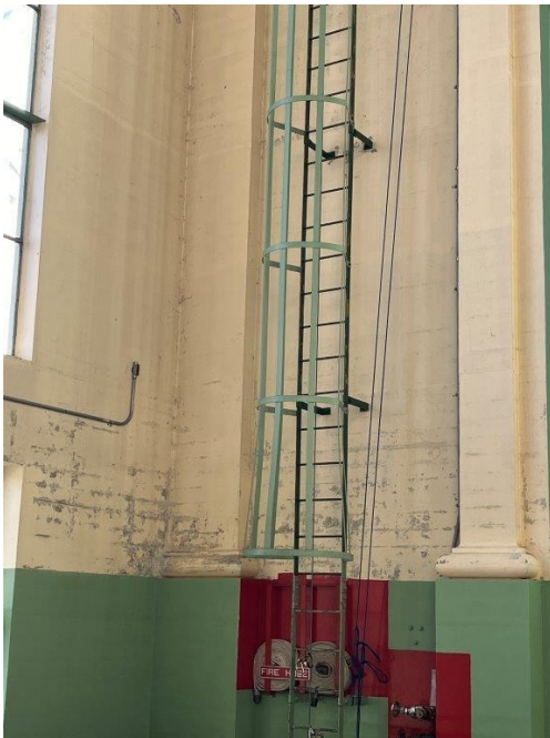
Access ladder to upper roof
