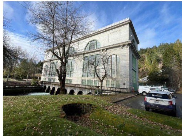
West view of Cushman 2 Powerhouse.
