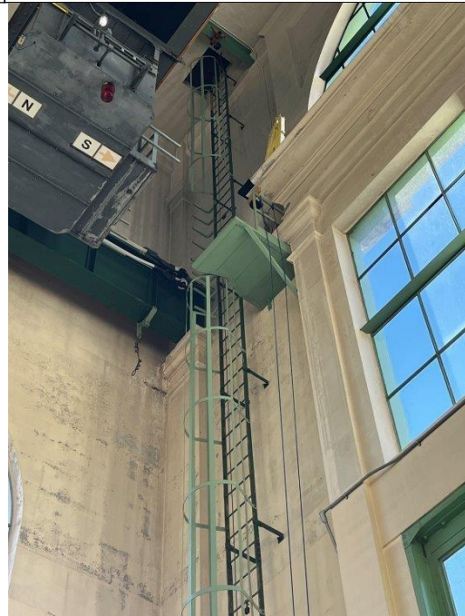
Access ladder to upper roof
