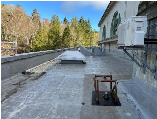
Annex roof looking north
