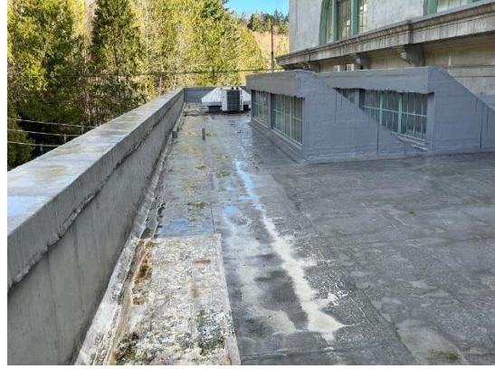
Annex roof looking north
