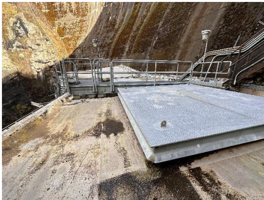
View of NF Powerhouse hatch covers, roof protrusions, walkway and connection of roofing material to the dam.
