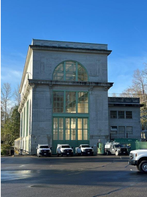
View SW of Cushman 2 Powerhouse. Upper roof to be reroofed, Annex to be reroofed and awnings upper and lower to be reroofed.
