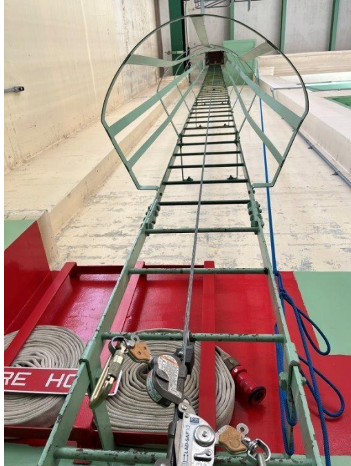
View of roof access
