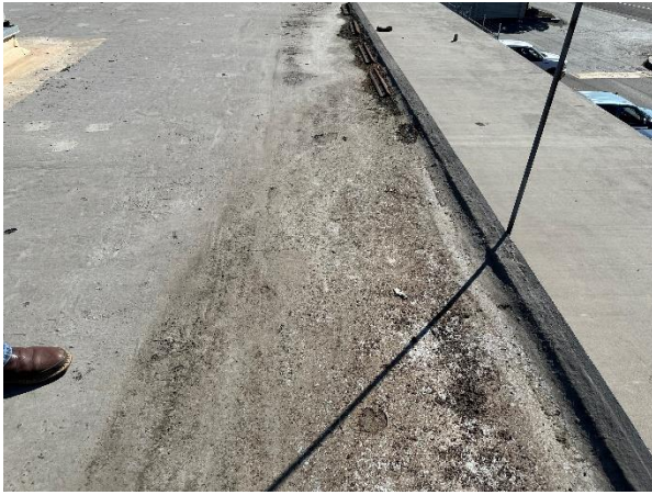
Edge of roof 1 looking east with roof 3 below.
