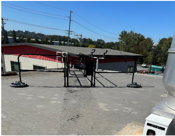
Roof 1 looking Southwest showing the attached walkway, roof 7 in the background
