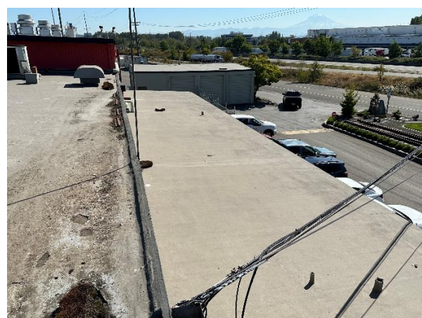
View of roof 1 edge and view of roof 6 below.
