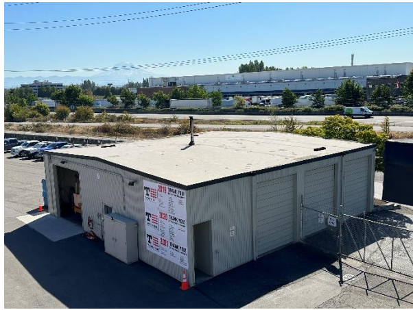
Maintenance building Roof 8
