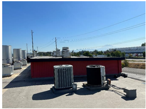
View looking east roof 1, roof 5 in the background
