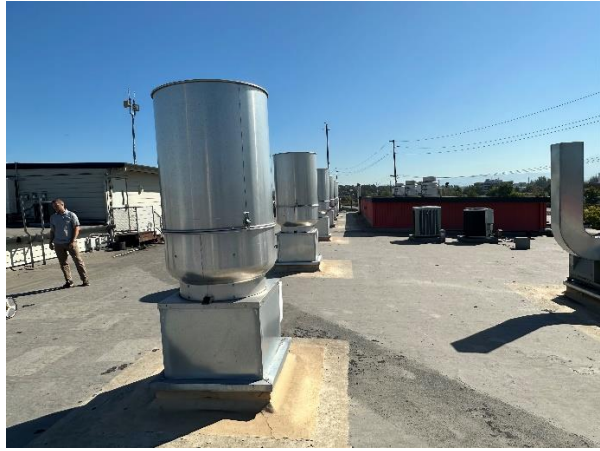
Roof 1 looking east, roof 2, roof 3 and roof 5 in the background
