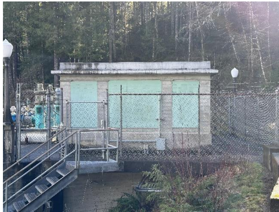
Intake house roof
