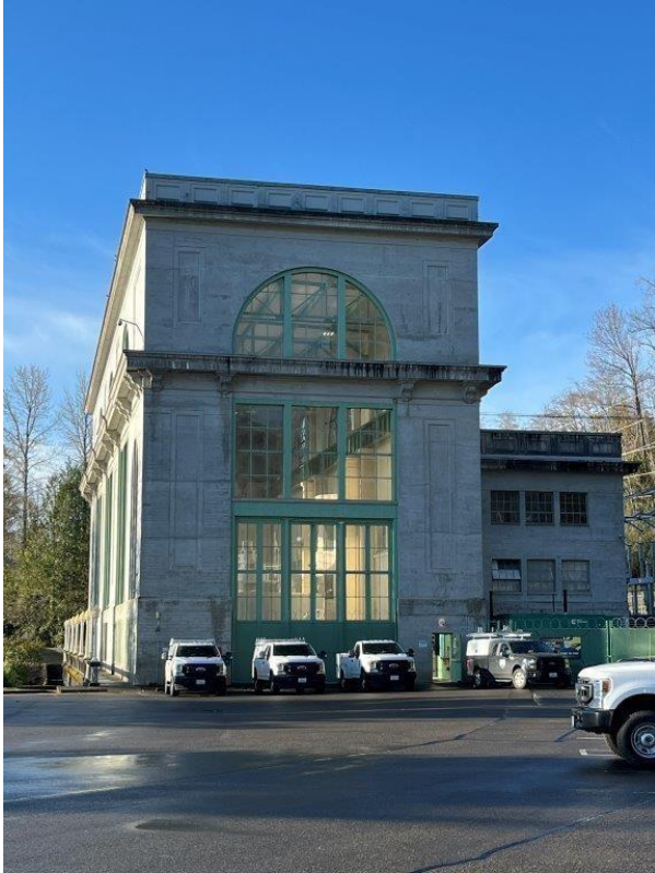
View SW of Cushman 2 Powerhouse. Upper roof to be reroofed, Annex to be reroofed and awnings upper and lower to be reroofed.
