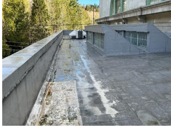
Annex roof looking north
