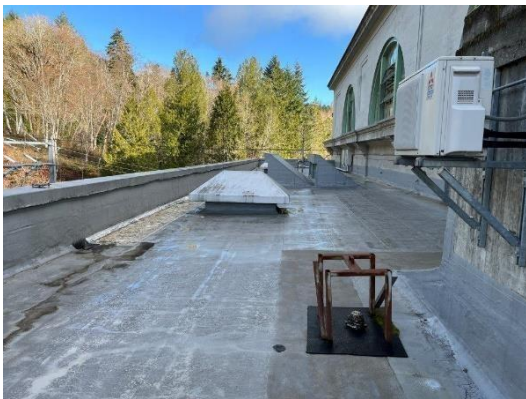
Annex roof looking north
