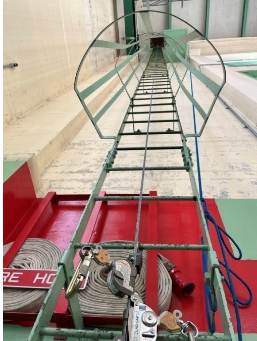
View of roof access
