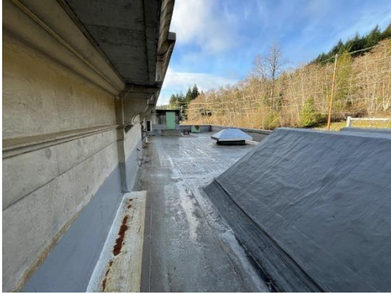
Annex roof looking south
