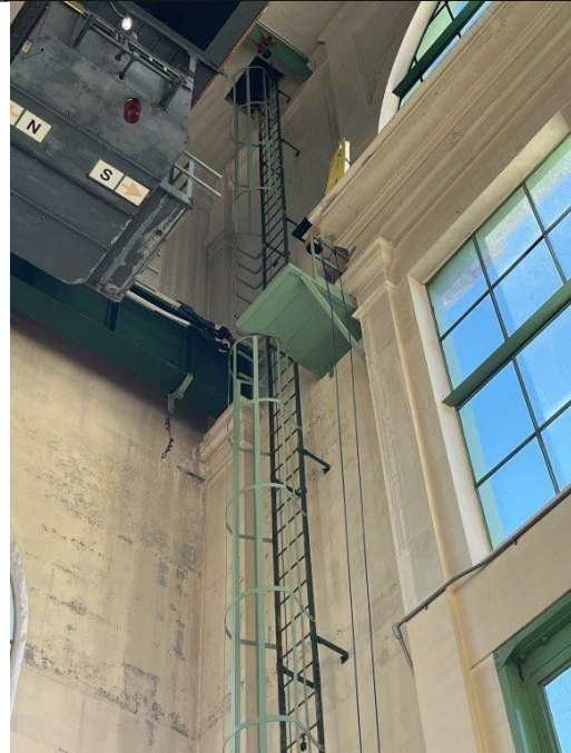
Access ladder to upper roof
