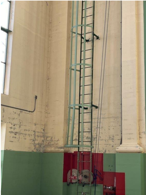
Access ladder to upper roof
