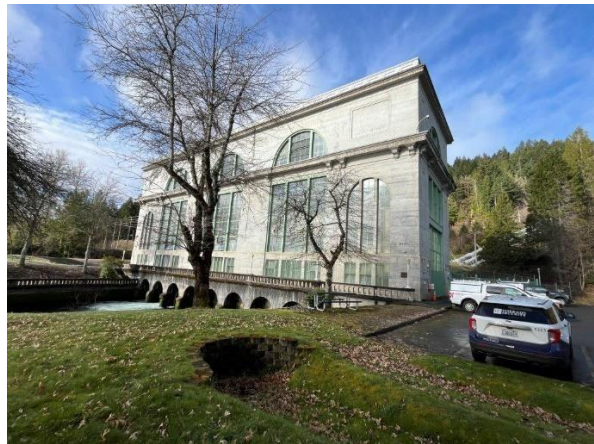
West view of Cushman 2 Powerhouse.
