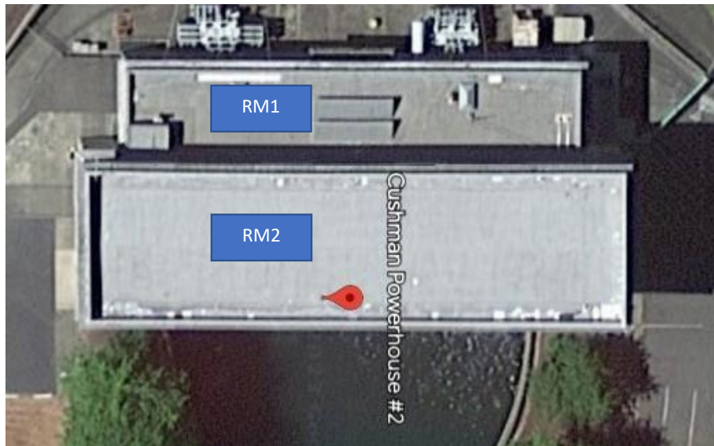
Roofing Locations taken from Cushman Powerhouse #2
