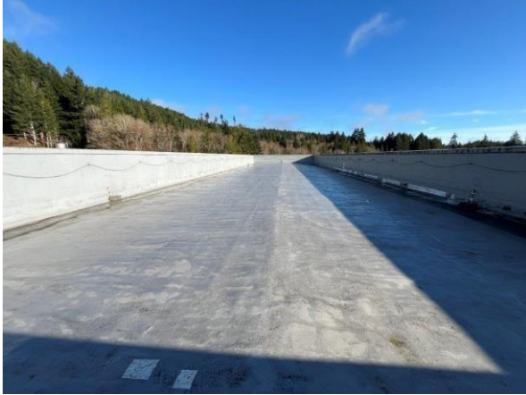
View SW of Cushman 2 Powerhouse. Upper roof to be reroofed, Annex to be reroofed and awnings upper and lower to be reroofed.
