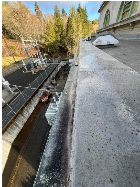
Annex roof overhang and roof vent
