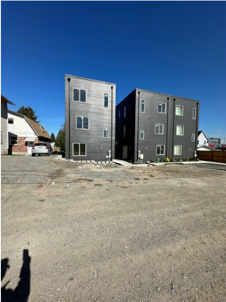
Parking at 1434 and 1436 are not paved.
