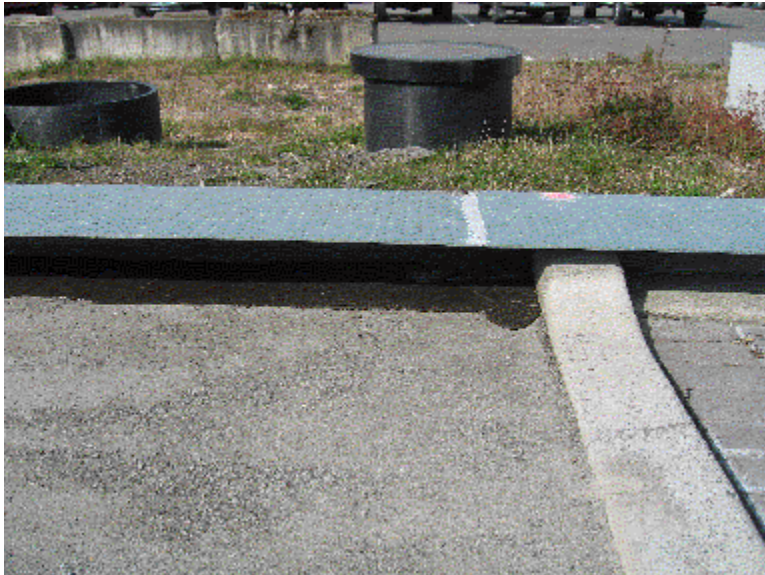
Figure 7-5b –Sampling Manholes and Curbing
